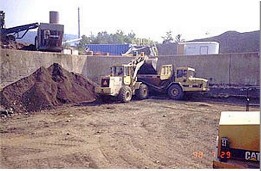
Loading treated soil for transport to onsite landfill.
