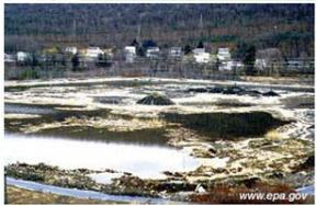
Landfill condition, February 1998, prior to the start of remedial action. Note water ponded on landfill surface.
